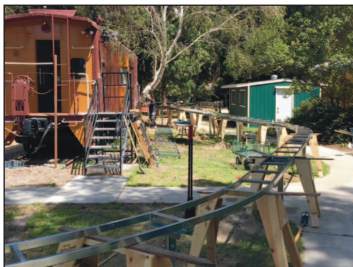
Custom steel framework comes together circumnavigating the SP bay window caboose.
