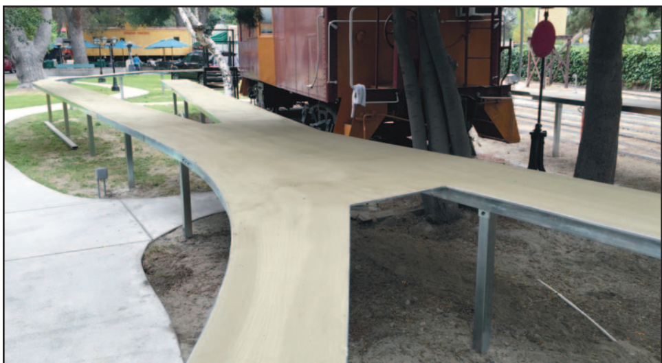
Heavy duty backerboard painted in sand-colored stucco provides a rugged surface for track.
