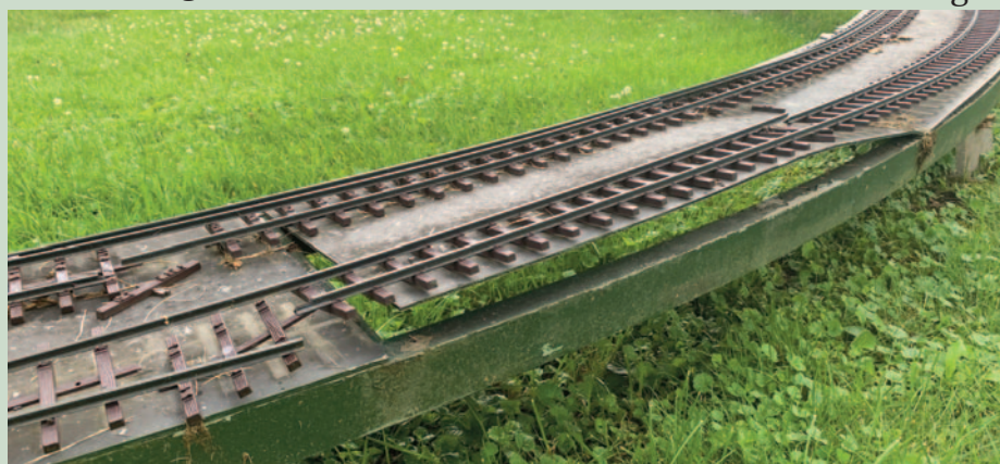
Above: An errant lawn mower caught the edge of the trackbed, bending the aluminum composite material and attached track, and ripping the rails from the ties. — Marie Brown Photo
